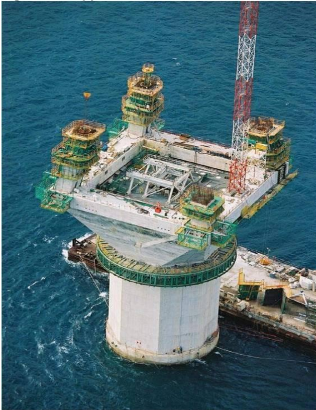
Figure 12: A pylon view
