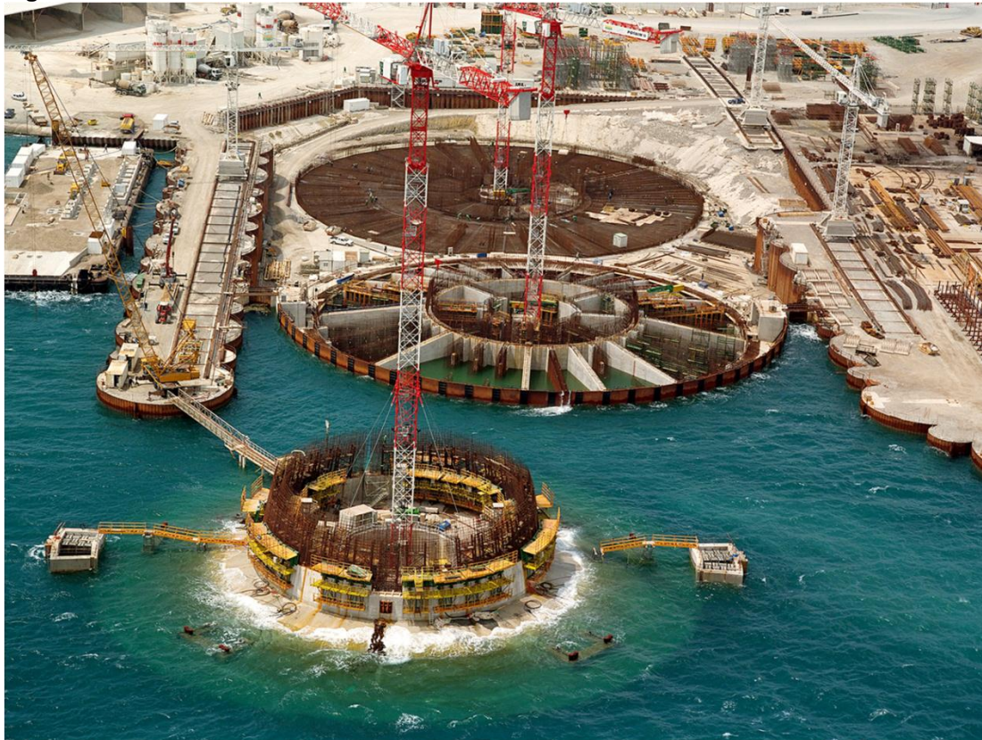
Figure 11: Placement of the first two fundamental bases
