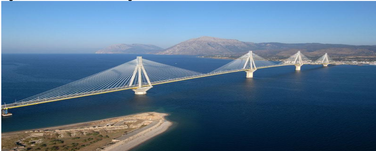
Figure 1: The Rion-Antirion Bridge
