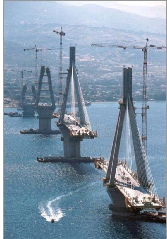
Figure 13: Deck installation
